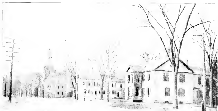
VIEW OF MAIN STREET, THOMASTON
